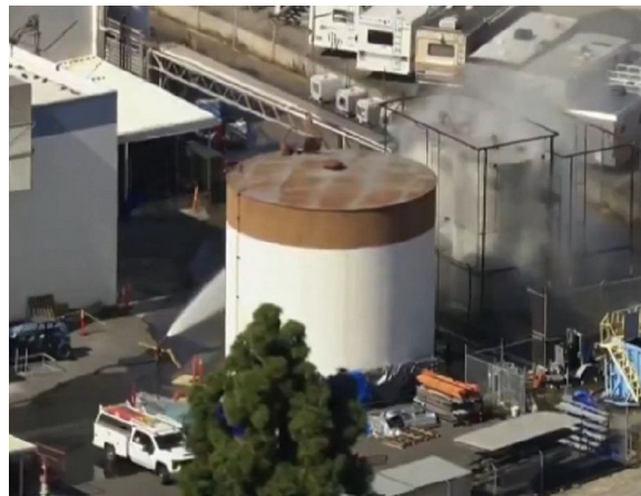
Crews cooling the overheating MMA tank.
