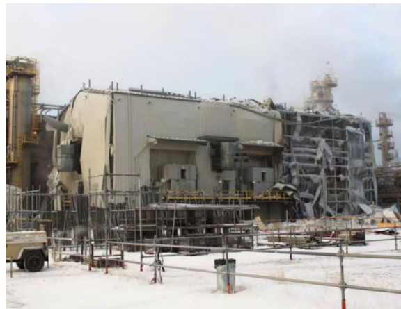
The hydrogen compressor building after the blast.
